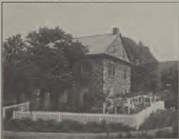
This stone house, a fine Pennsylvania example of the Georgian style has been erroneously called the oldest in the borough. It was built about 1803 on the farm of Jacob Ehbrenhardt, one of the founders of the village, presumably by his only son Jacob (1760-1825). Then it was not within the village confines; today it is on South Keystone Ave., just beyond the East Penn Railway.
